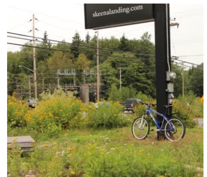
A lack of bicycle parking can result in cyclists locking up to a variety of features
