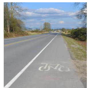
Recent shoulder widening on the approach to the Old Bridge on Highway 37 (top); pavement stencils in a rural paved shoulder (below).
